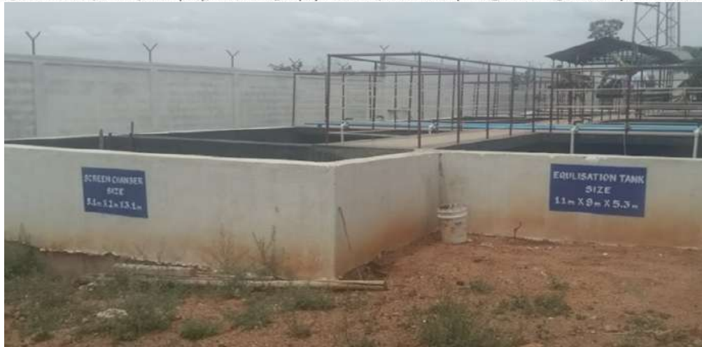
Figure 4: Equalization Tank (5 KLD)
