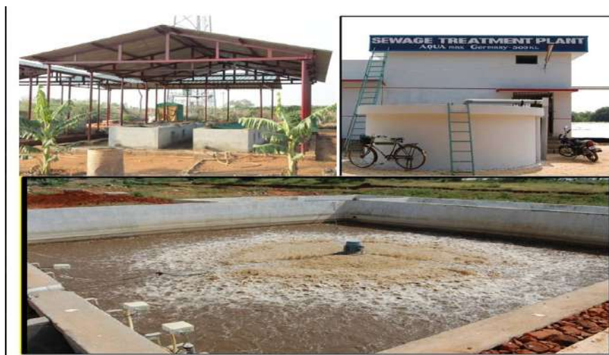
Figure 5: Sewage Treatment Plant 300 kld
