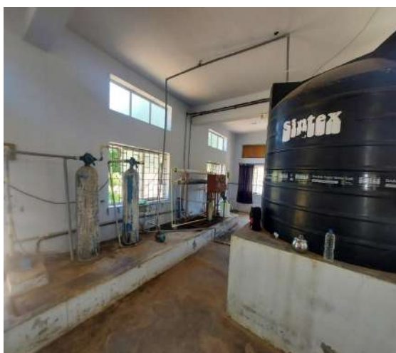
Figure:3 Reverse Osmosis Plant (Old & New)
