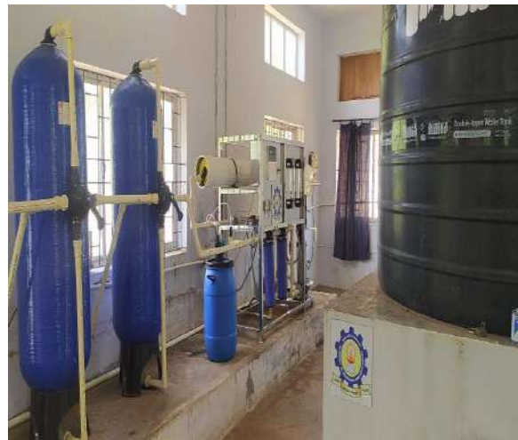
Figure:3 Reverse Osmosis Plant (Old & New)
