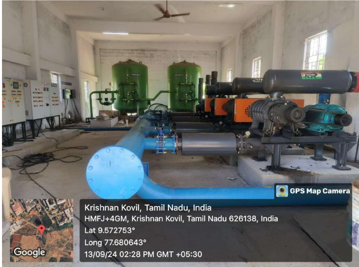
Figure: 9 Tertiary treatment of sewage water using rapid sand filter, activated charcoal, UV and Chlorine disinfection
