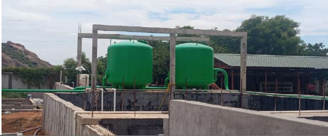
Tertiary treatment of sewage water plant
