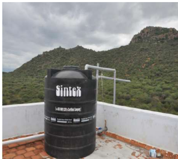
Figure:4 Dual Pipeline system used for treated water
