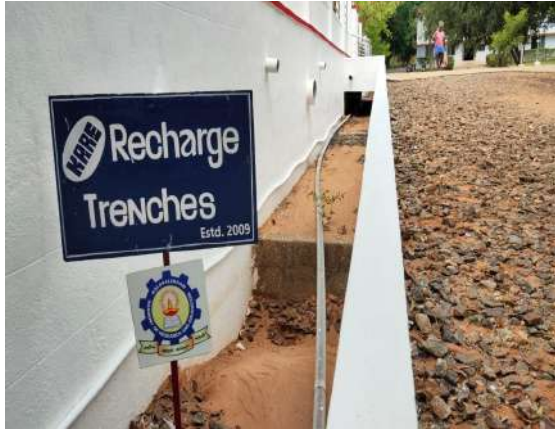
Figure:2 Recharge Trenches & Percolation Ponds at KARE
