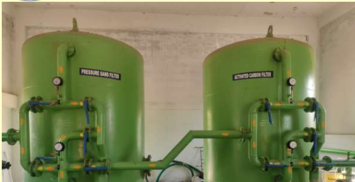
Adsorption Column (Rapid Sand Filter and Activated Charcoal Filter) Facility in the STP at Kalasalingam Academy of Research and Education.
