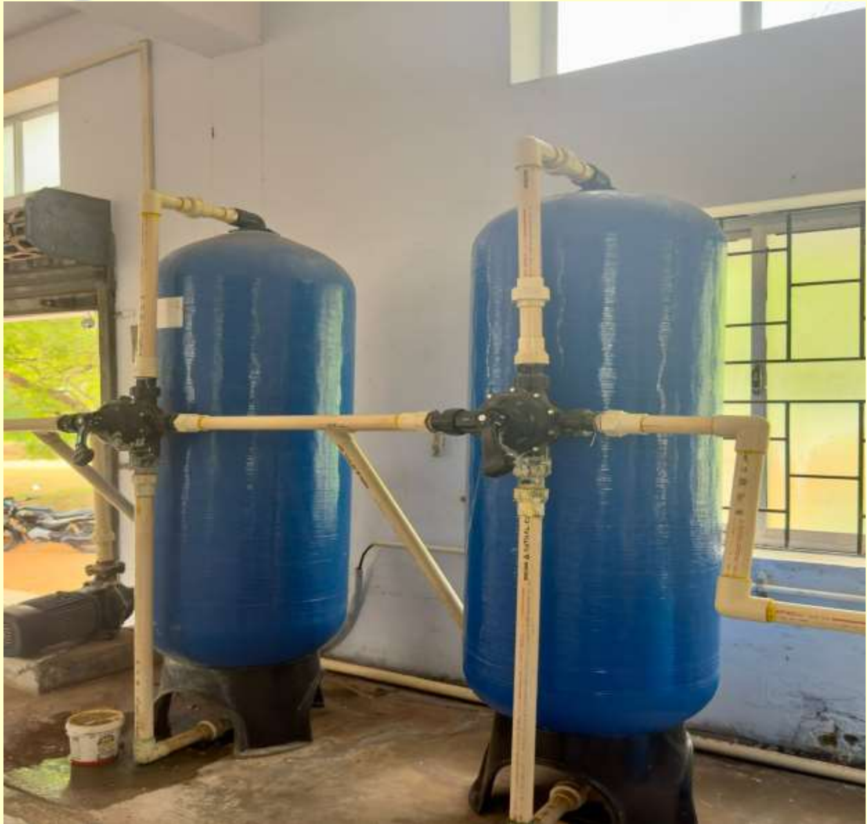
Multi graded filter in Mineral water treatment plant
