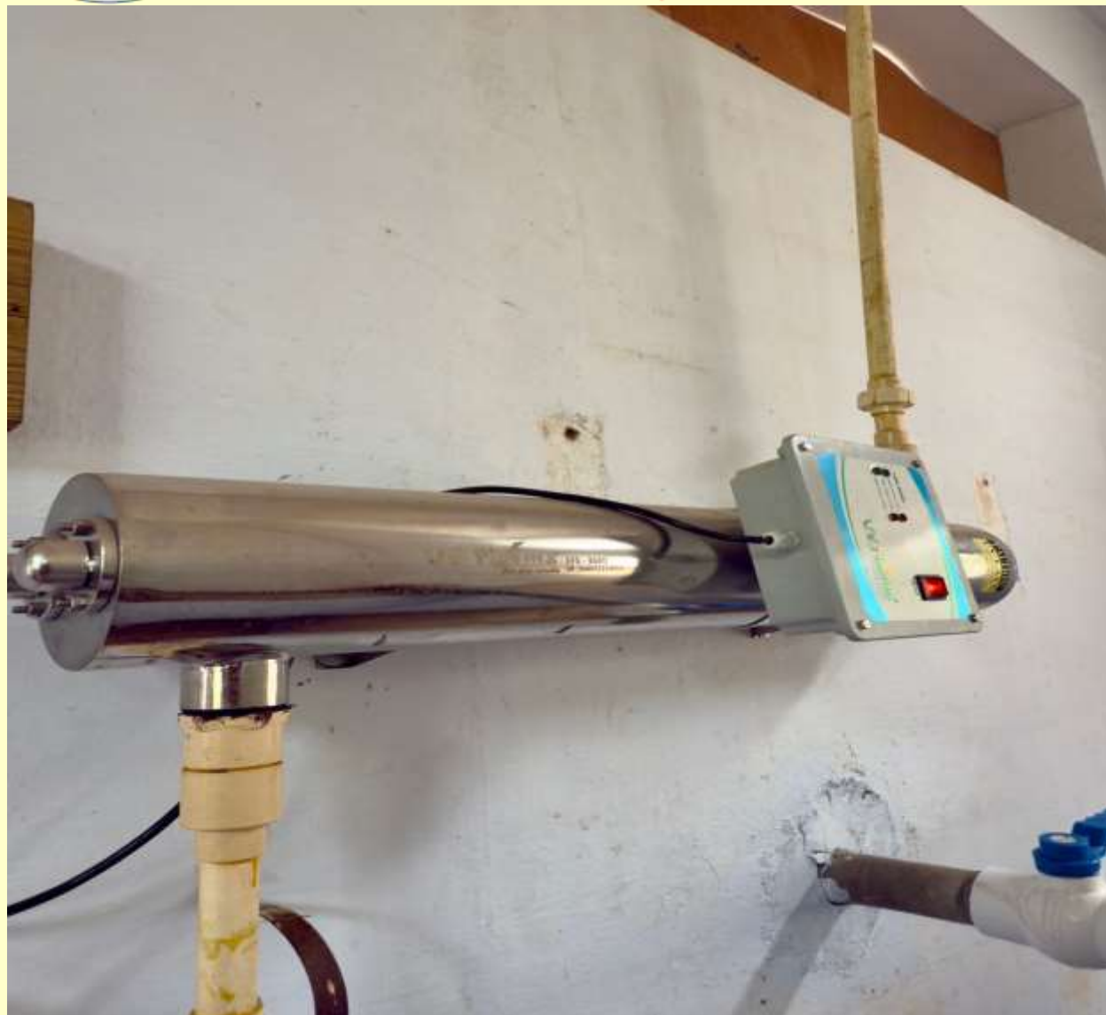
Disinfection of Water with UV Treatment
