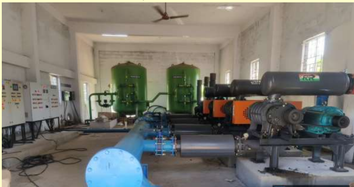
Adsorption Column (Rapid Sand Filter and Activated Charcoal Filter) Facility in the STP at Kalasalingam Academy of Research and Education.
