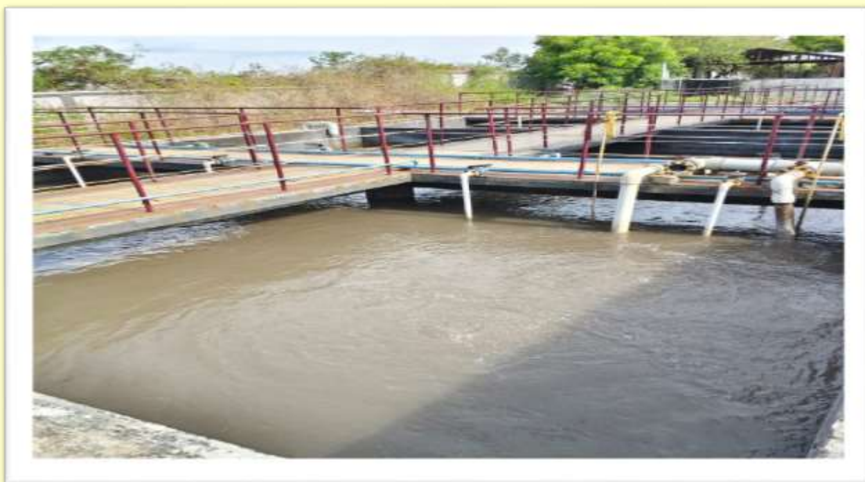
Aeration to the Wastewater in Sequential Batch Reactor
