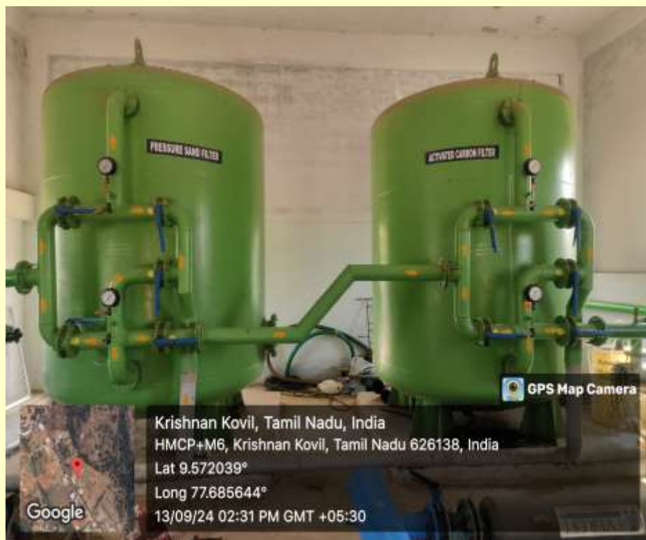
Adsorption Column (Rapid Sand Filter and Activated Charcoal Filter) Facility in the STP at Kalasalingam Academy of Research and Education, TN
