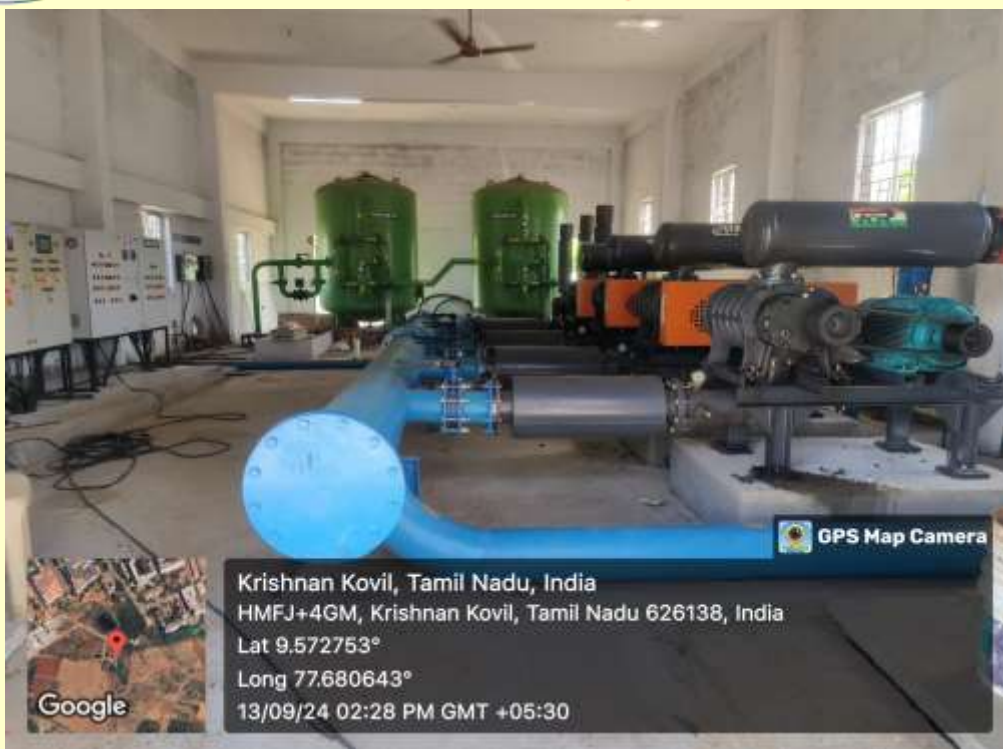
Air Blower Pumps Facility in the STP at Kalasalingam Academy of Research and Education, TN Sludge management
